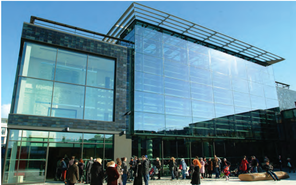
Jubilee Library, Brighton LCE Architects Ltd
